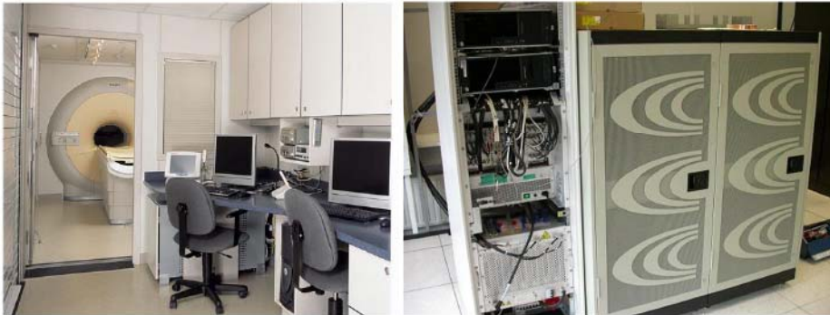
(a) Operator Room
